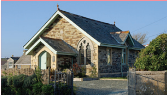
This example of a domestic conversion at Trevone near Padstow shows how new uses can retain the distinctive quality and character of chapels in their settings. Most chapels will be conserved through this form of reuse. Photo © Eric Berry
