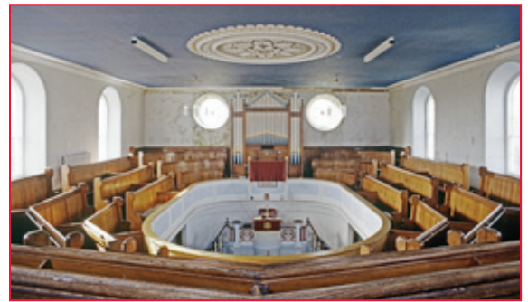
The interior of the 1862 Wesleyan chapel at Leedstown in Crowan parish (grade II) has an original gallery. However, as with so many Methodist chapels, the building was re-seated in the late 19th century with simple pitch pine pews. Photo © Eric Berry
