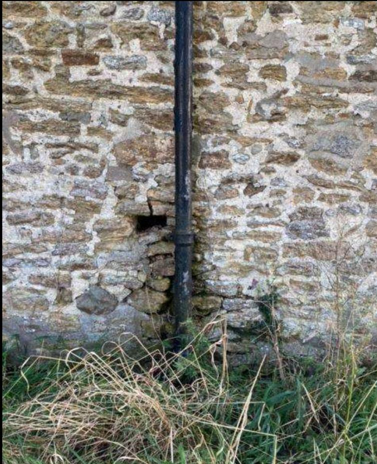
The old boiler flue has left a gap in the wall and a dangerous 'pit' in the churchyard.
