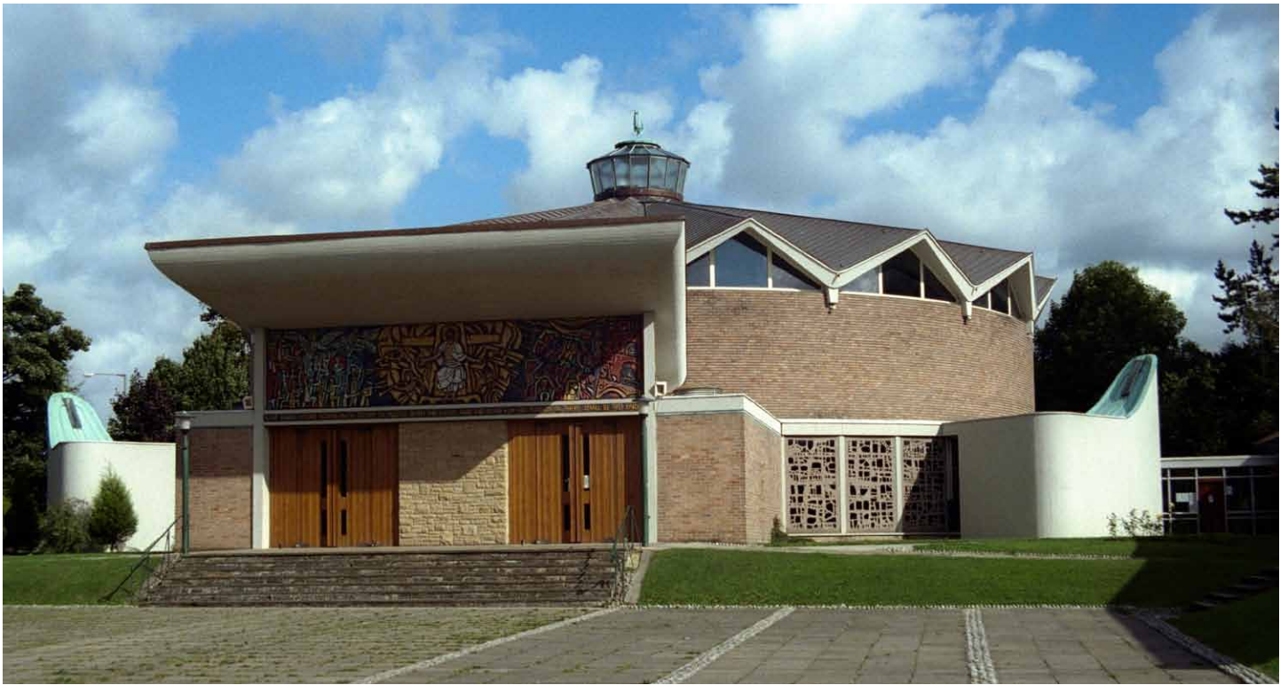
Fig 12. Built with a central altar, and on a circular plan, the Roman Catholic church of St. Mary, Leyland (Lancashire), of 1962-4, is an embodiment of the shift in liturgical practice following Vatican Council II. Designed by Weightman and Bullen, it is listed Grade II.
