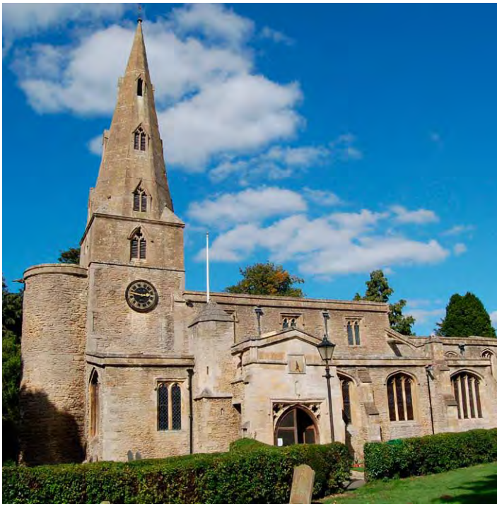
Fig 2. St. Andrew's, Brigstock, Northamptonshire. This village church is typical in that its long and complex structural history is readily apparent. That evidences architectural fashions and also, importantly, evolving liturgical requirements. The tower, including the rounded stair turret, is late Anglo-Saxon. Listed Grade I.
