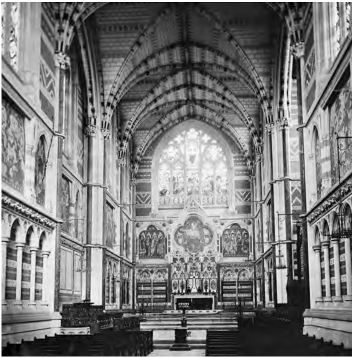
Fig 8. One of the most significant religious buildings of the Gothic Revival, the Chapel of Keble College, Oxford, with its polychromatic brickwork and expansive plan, set the model for many urban churches of the second half of the nineteenth century. Designed by William Butterfield in 1876, he declared he had a 'mission to give dignity to brick'. Photograph of the interior taken in 1880. Listed Grade I.
