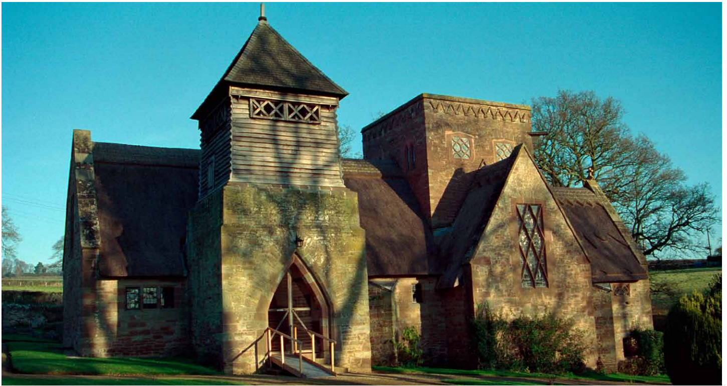
Fig 10. Something of a technological wolf in sheep's clothing, the traditional thatch of All Saints', Brockhampton, Herefordshire, disguises a concrete roof. Designed by the Arts and
