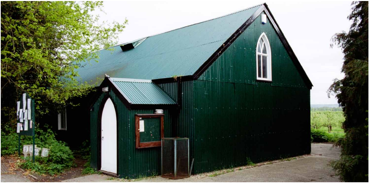
Fig 11. 'Tin Tabernacles' were pre-fabricated, corrugated iron-clad churches erected from the mid nineteenth century. They served fast-growing urban areas, while permanent churches were being built, as well as remoter settlements or new faith groups. Now often in other uses this 1914 example, the Golden Green Mission church in Hadlow, Kent, is now an uncommon survivor. Listed Grade II.
