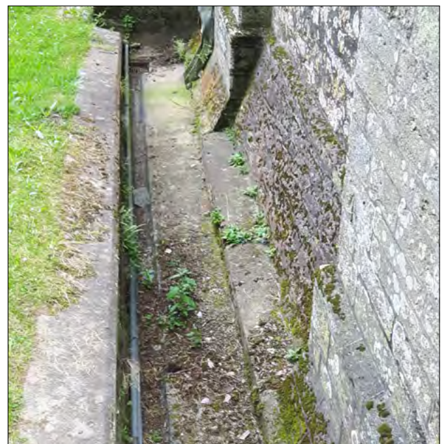
St Germans Priory's surface drainage / gully
