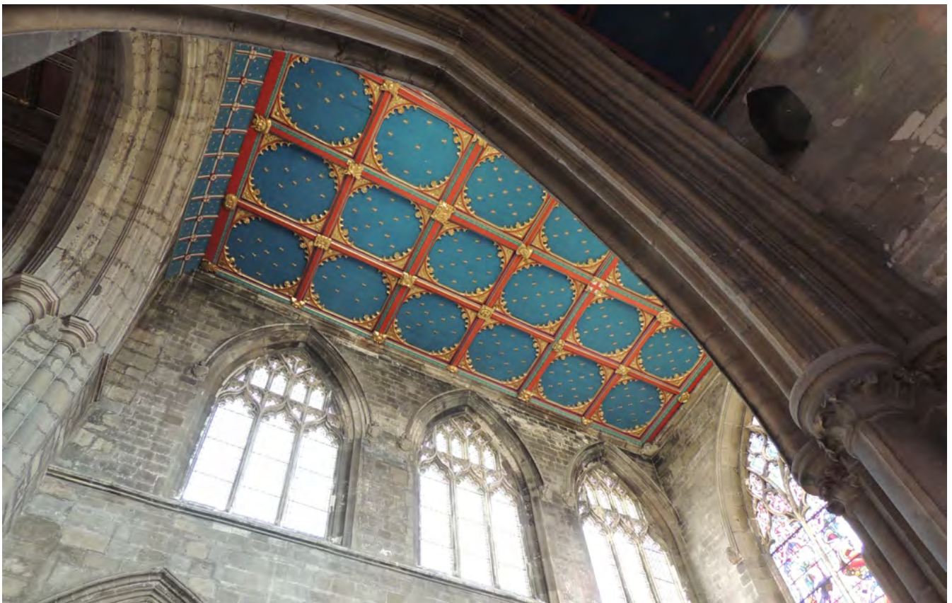
Nave ceiling at St Mary's © St Mary's PCC
