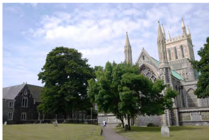
Great Yarmouth Minster (east end) within its setting of churchyard and priory buildings
