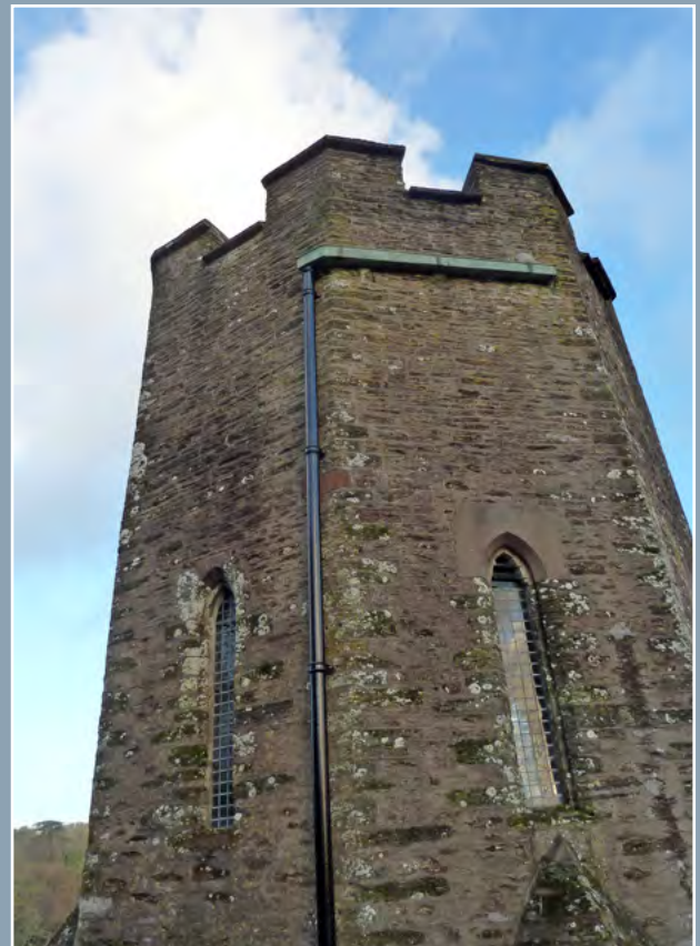
Replaced downpipes on the north-west tower © Le Page Architects
