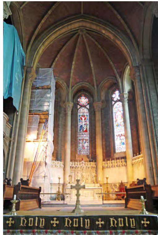
View of the sanctuary
