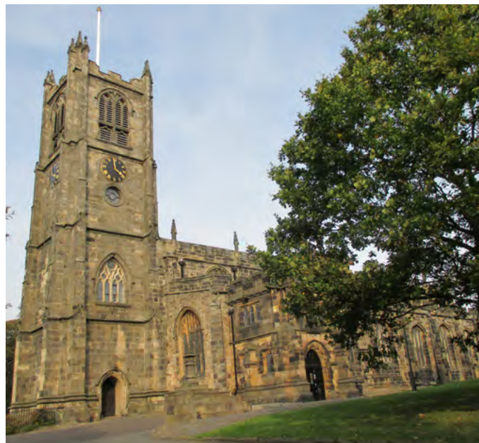
Lancaster Priory, exterior - Antiquary - Own work - File:Lancaster Priory 2.JPG - CC BY-SA 4.0 [ http://creativecommons.org/licenses/by-sa/4.0/ ]
