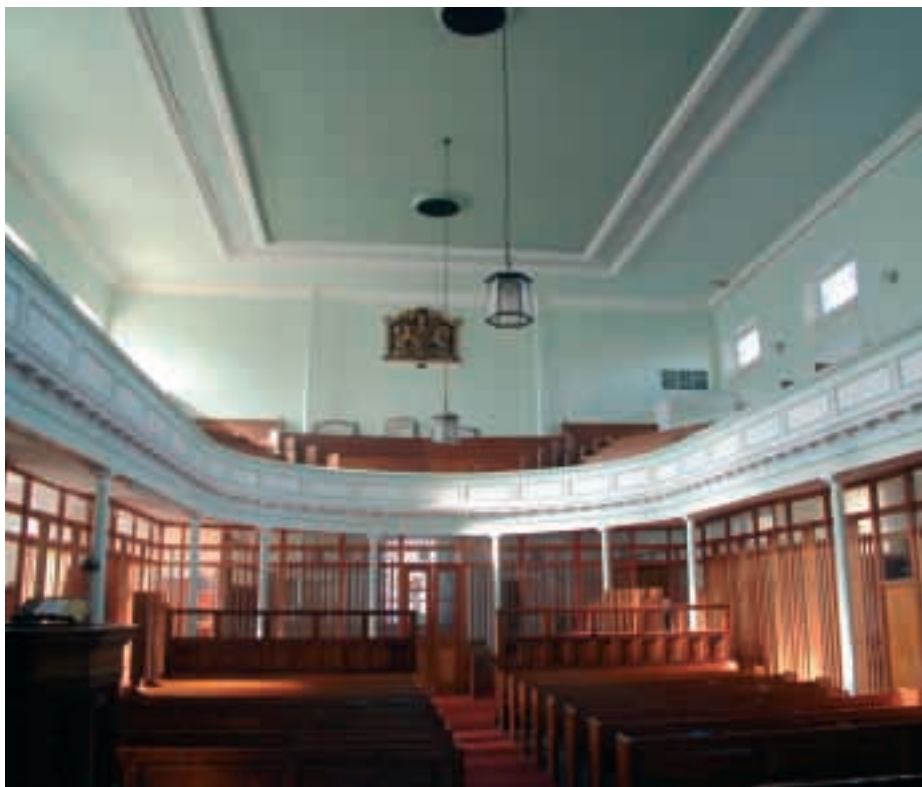
Figure 6 Enclosing the space beneath galleries can create additional separate rooms.
