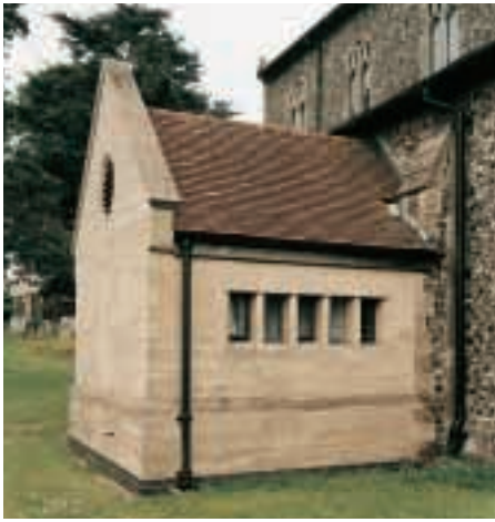
Figure 8 Constructing a porch-like addition to this church has provided a lavatory and small kitchen.
