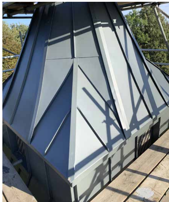
Photo: Zinc covering on a church spire © Bakers of Danbury
