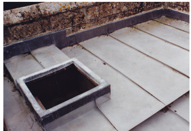
Figure 4: Lead used for flashings and access hatch capping
