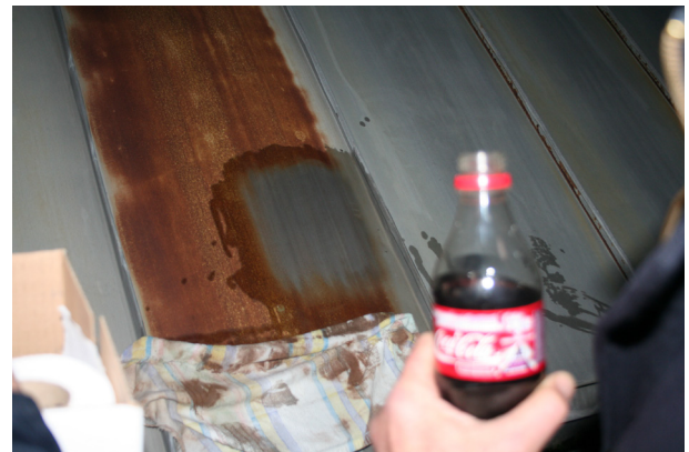
Figure 10: Stain successfully removed using weak phosphoric acid solution
