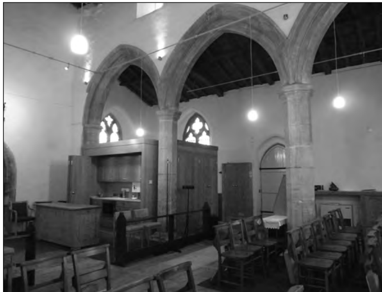
Fig. 2: St Mary, Orton Waterville, Cambridgeshire. A 'pod' has been inserted at the west end of the north aisle with a kitchen area, storage and toilet
