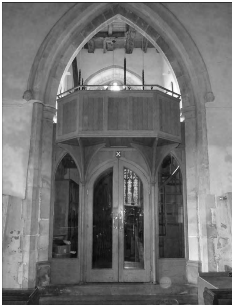
Fig. 3: St Andrew, Oakington, Cambridgeshire has filled up the base of the west tower with facilities
