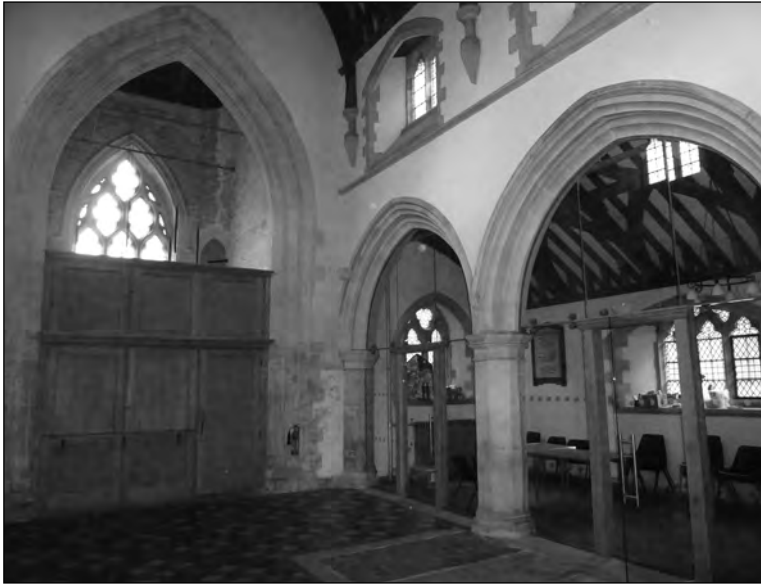
Fig. 4: St James, Stretham, Cambridgeshire. The church has used glass screening to create a meeting room in the north aisle and used the base of the tower for a kitchen and toilet
