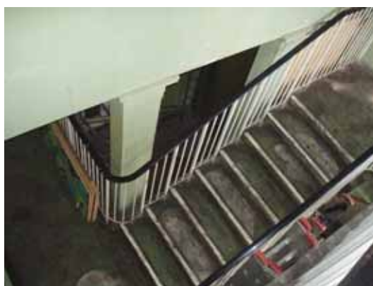
North west staircase (now a fire escape), 2006
