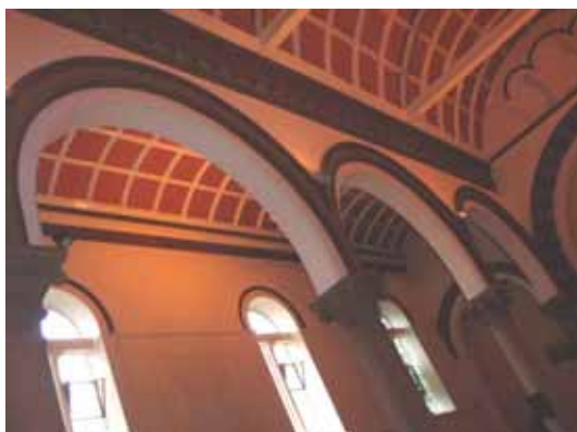
G.E. Street's nave arcading (1871-2)
