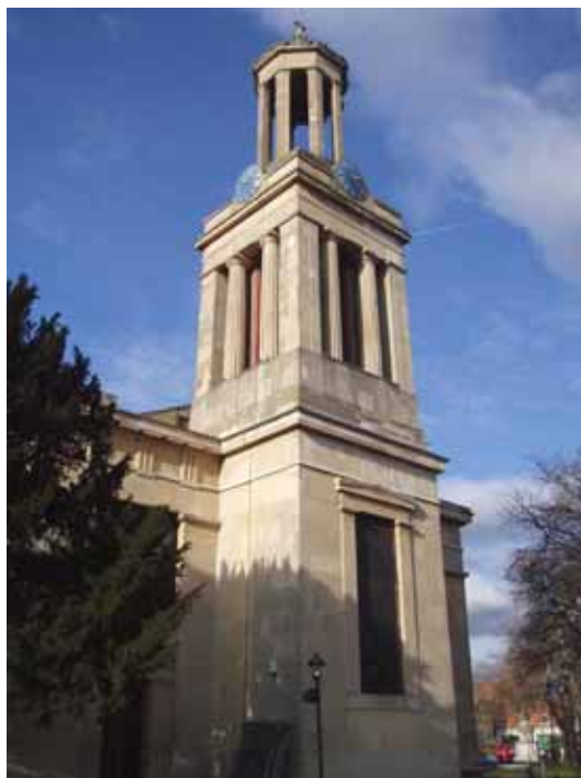
Church tower to east end of church, 2006
