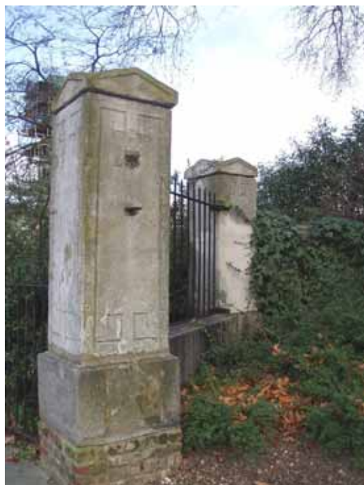
Gateposts and railings to south west of west front, 2006
