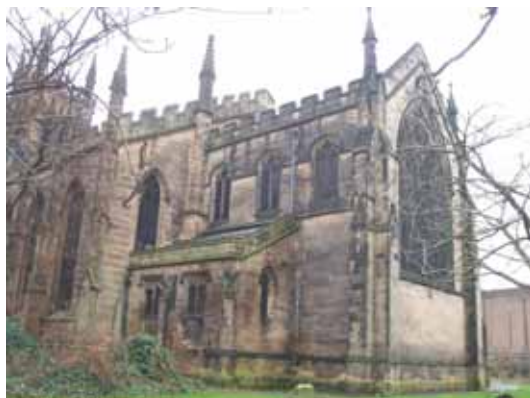
Chancel from south east, 2006
