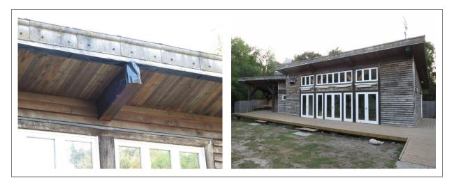
**Figure A1.3** – One-way exclusion measure installed at Studland. On buildings that have a large number of potential roost access points, plastic sheeting is a cheap material that can be used to seal off large parts of the building while leaving simple one-way measures at key exit points (identified during emergence surveys). Images: Matt Zeale
