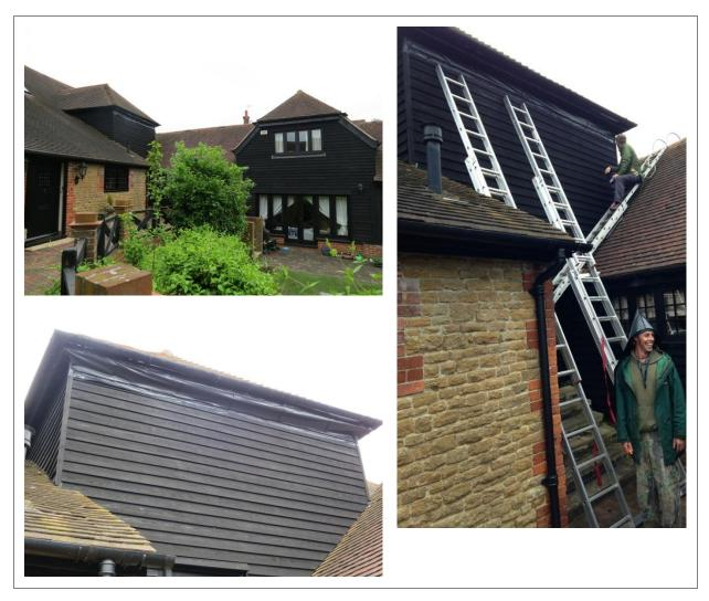
**Figure A1.2** – One-way exclusion measure installed at Shackleford. Plastic 'flashing' can be used to great effect to exclude bats from roosts where multiple roost exits exist along the length of a building under eaves. Images: Matt Zeale
