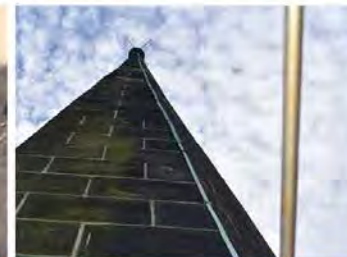
Lightning Protection System Inspection
