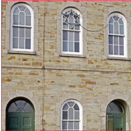
Panelled doors with fanlights and hornless sash windows, as exemplified within the 1860 pedimented façade of the Wesleyan chapel at St Agnes (grade II). Photo © Eric Berry
