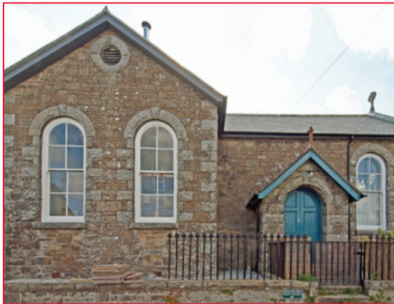
Horned sash windows are marked by projecting lugs, which help to strengthen the meeting rails in combination with the heavier glass used from the mid 19th century. They are a type commonly used from the 1870s in Cornwall. This is the (unlisted) late chapel at Newbridge in Sancreed parish. Photo © Eric Berry
