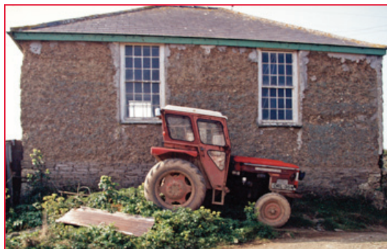
The 1838 former Free Methodist chapel at Tregona (grade II) in St Eval parish is a good vernacular example with cob (earth) walls on stone rubble footings. Photo © Eric Berry
