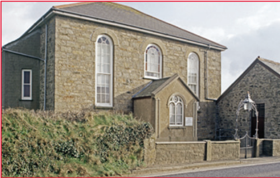
The rather unusual mid-19th century chapel at Trewennack in Wendron parish has round-arched sash windows set into stone rubble walls. The roadside elevation was fitted with a later central entrance porch so that the later Sunday School (right) was accessed from the roadside forecourt. Photo © Eric Berry
