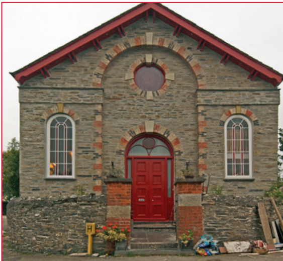
The gabled façade to this chapel (opened 1874) at Tredrizzick has a recessed central bay rising to an open pediment. Its show front, with the central bay and entrance picked out in coloured brickwork, is almost identical to that of the 1869 chapel at St Tudy (grade II). Photo © Eric Berry
