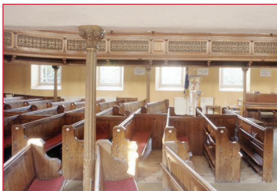
The interior of the 1858 unlisted chapel at Bugle was completely remodelled and refitted in 1890. The pitch-pine pews are of a standard design with v-jointed boards and shaped ends with ceramic numbers but the richly decorated panelled and pilastered gallery front is emphasised by its architectural treatment. Photo © Eric Berry
