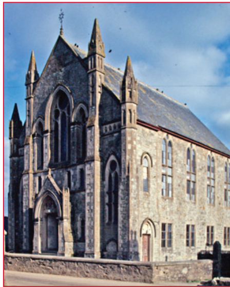
This late-19th century chapel at Perranwell exhibits the key distinguishing features of many Gothic chapels – a focus on the façade, the functional side elevations betraying the existence of galleries, and references to an earlier Picturesque Gothic style in its use of finials topping the buttresses on the façade. © Eric Berry
