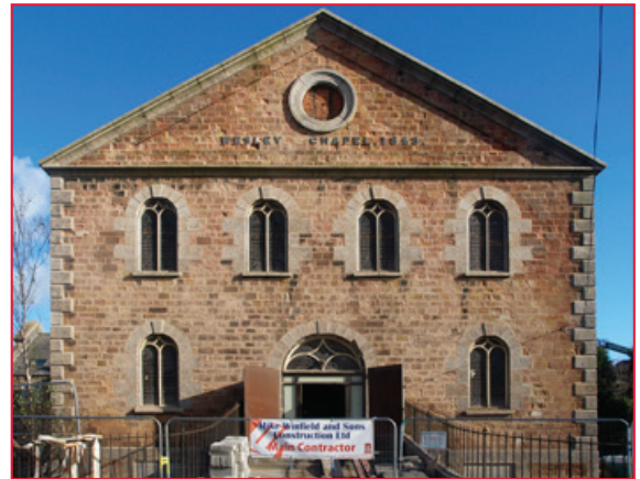
By the end of the 19th century windows were being installed with paired lights and a roundel, either in a pointed-arched or round-headed opening. These windows were inserted within the original openings of the 1843 (grade II) Classical chapel at Tuckingmill. Photo © Eric Berry
