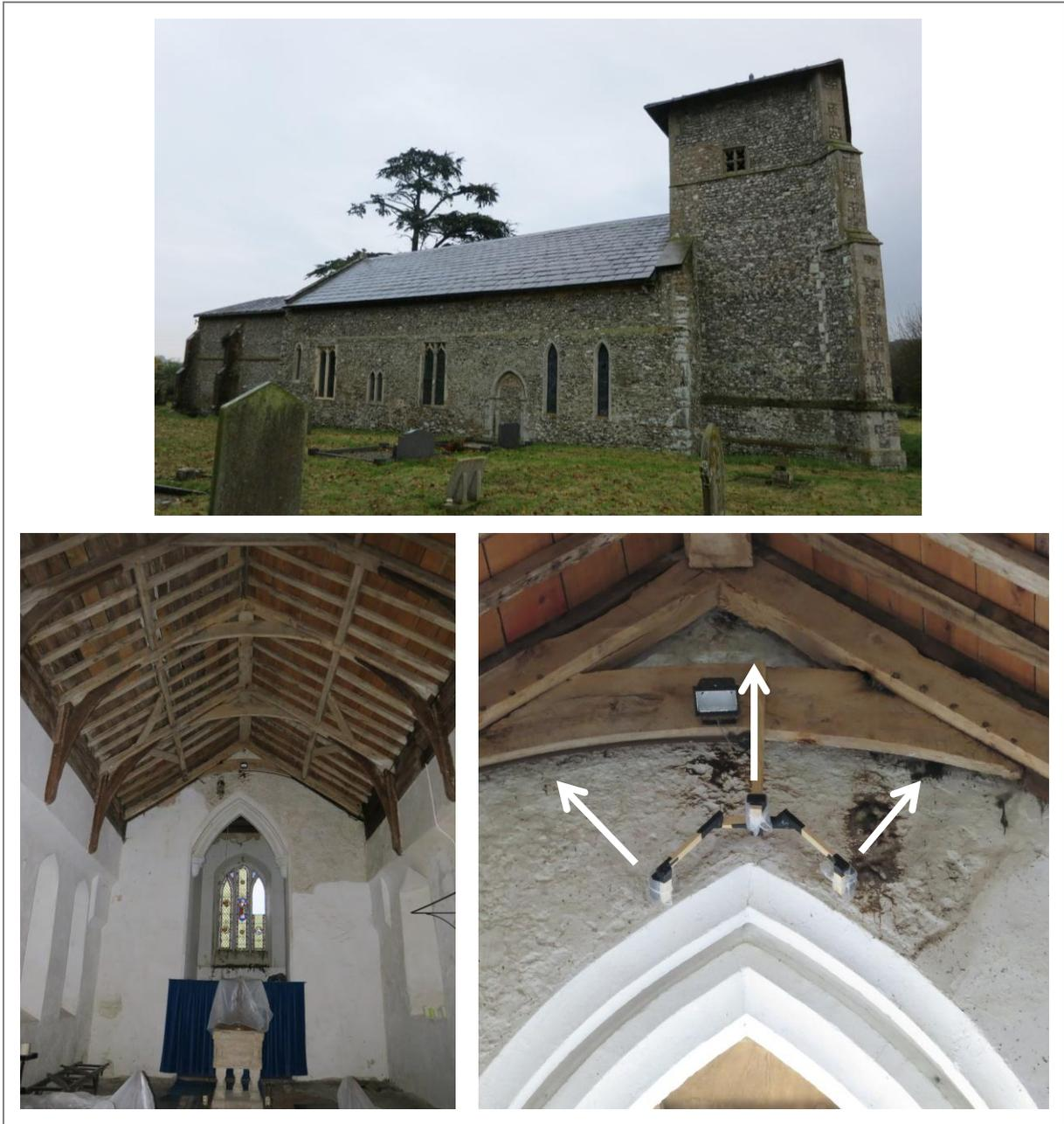
**Figure A6.2** – All Saints church at Toftrees. Shows (bottom right) three CR deterrent units mounted on a rig designed to broaden the directionality of the combined units. A colony of >100 Natterer's bats roost in among the mortise joints of the roof timbers. Note the staining on the wall from droppings and urine. Images: Matt Zeale
