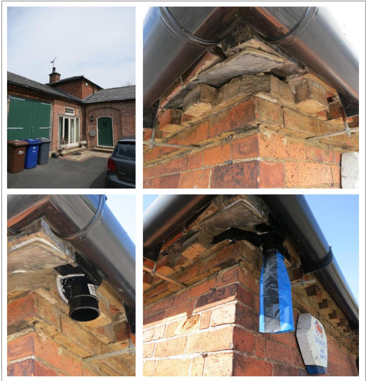
**Figure A1.1** – One-way exclusion measure installed at Crakemarsh. In this example, gaps in brickwork are filled in and one hole is left open to create a single exit point for bats. Plastic guttering and a plastic bag ‘shoot’ create an effective one-way exclusion measure for bats. Images: Matt Zeale
