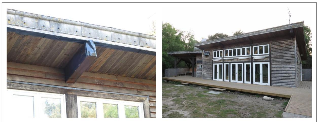
**Figure A1.3** – One-way exclusion measure installed at Studland. On buildings that have a large number of potential roost access points, plastic sheeting is a cheap material that can be used to seal off large parts of the building while leaving simple one-way measures at key exit points (identified during emergence surveys). Images: Matt Zeale
