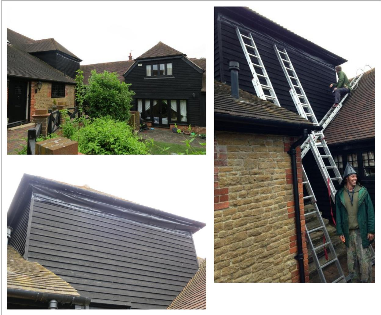
**Figure A1.2** – One-way exclusion measure installed at Shackleford. Plastic ‘flashing’ can be used to great effect to exclude bats from roosts where multiple roost exits exist along the length of a building under eaves. Images: Matt Zeale
