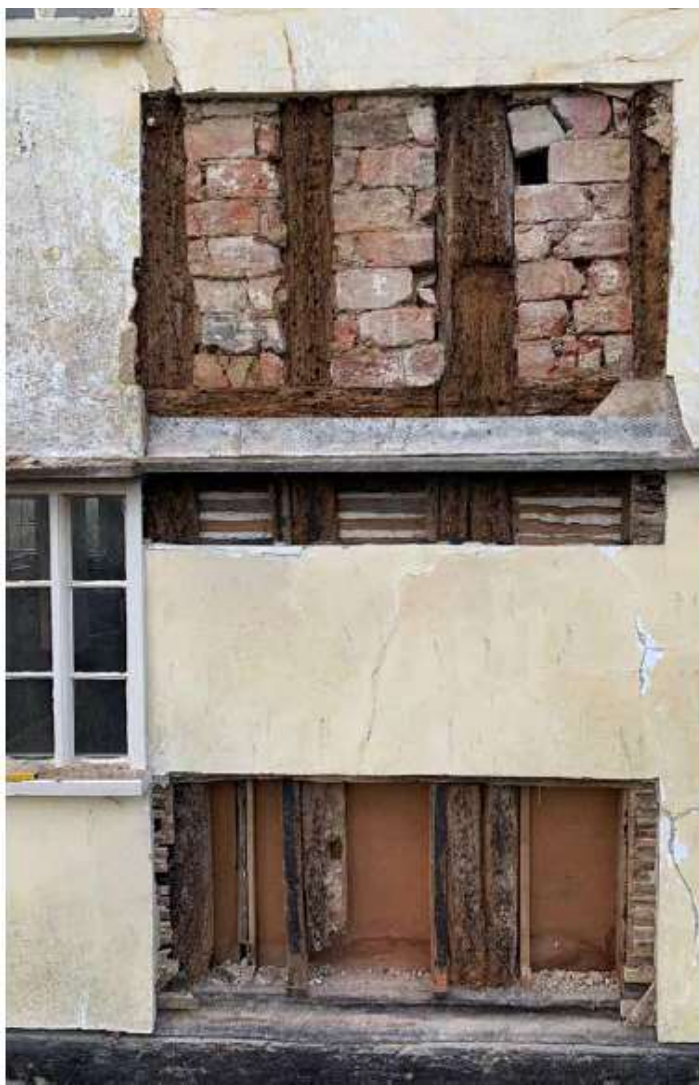
Figure 112. Example area of opening up on the East Elevation, showing the condition of the timber frame, surviving brick infill to the upper storey and no infill at all to the lower storey.
